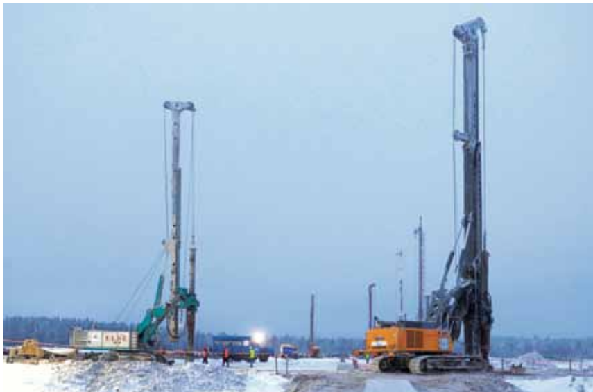
Portovaya compressor station construction
