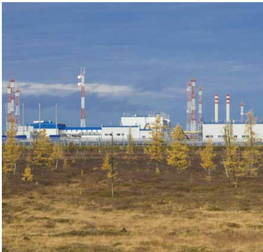
Comprehensive gas treatment unit No.22
