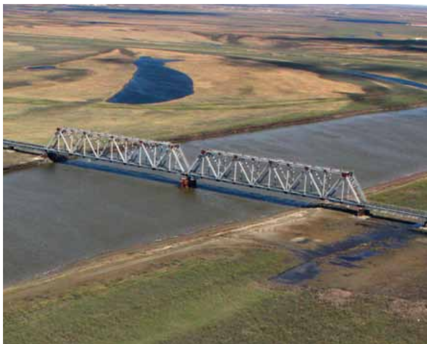
Yuribey River bridge crossing
