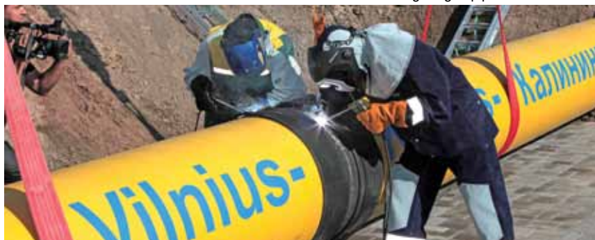
Minsk – Vilnius – Kaunas – Kaliningrad gas pipeline construction
