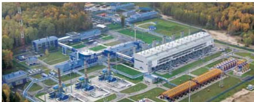
Voskresensk compressor station
