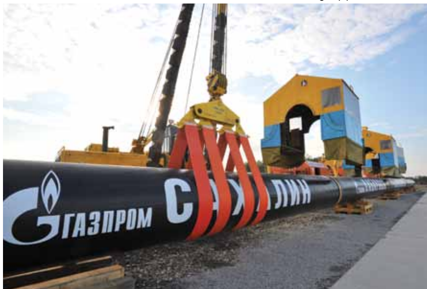
Sakhalin – Khabarovsk – Vladivostok gas pipeline construction
