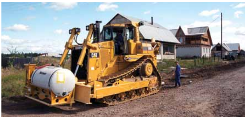
Inter-settlement gas pipeline placement
