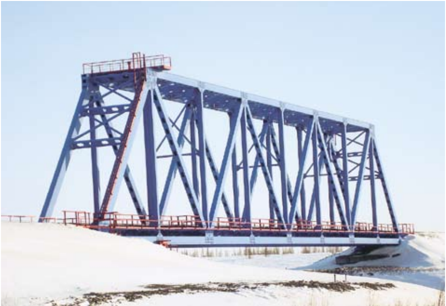
One of the 37 Bridge Crossings at the Obskaya – Bovanenkovo Railroad
