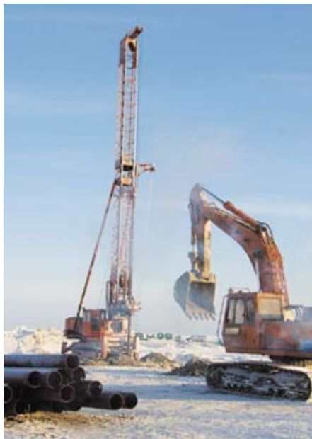
Pre-Development of the Bovanenkovskoye field is progressing in full swing
